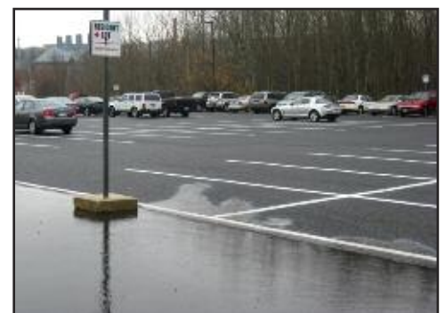
Porous asphalt parking lot on the UConn campus, during a rain storm. Note the runoff on the conventional asphalt in the foreground. Photo by C. Bellucci, CT DEP.
